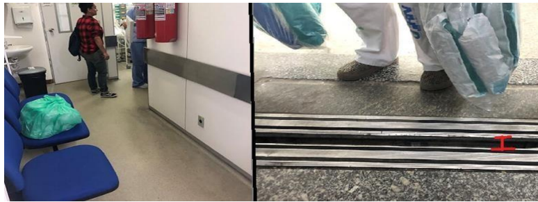
Figure 4. Access to Maternity Unit A and elevator elevation. (Authors, 2019)
