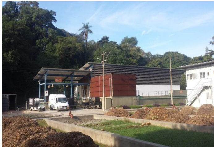
Figure 8 Fiocruz Hazardous Product Waste Deposit Area
